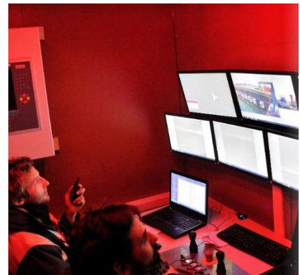
Figure 2 The control room
